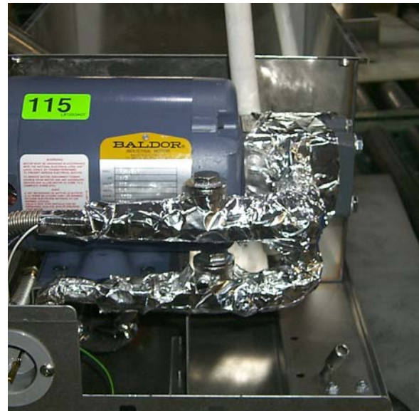
Heater strip installed [115V PF50 (Return/Suction)].
